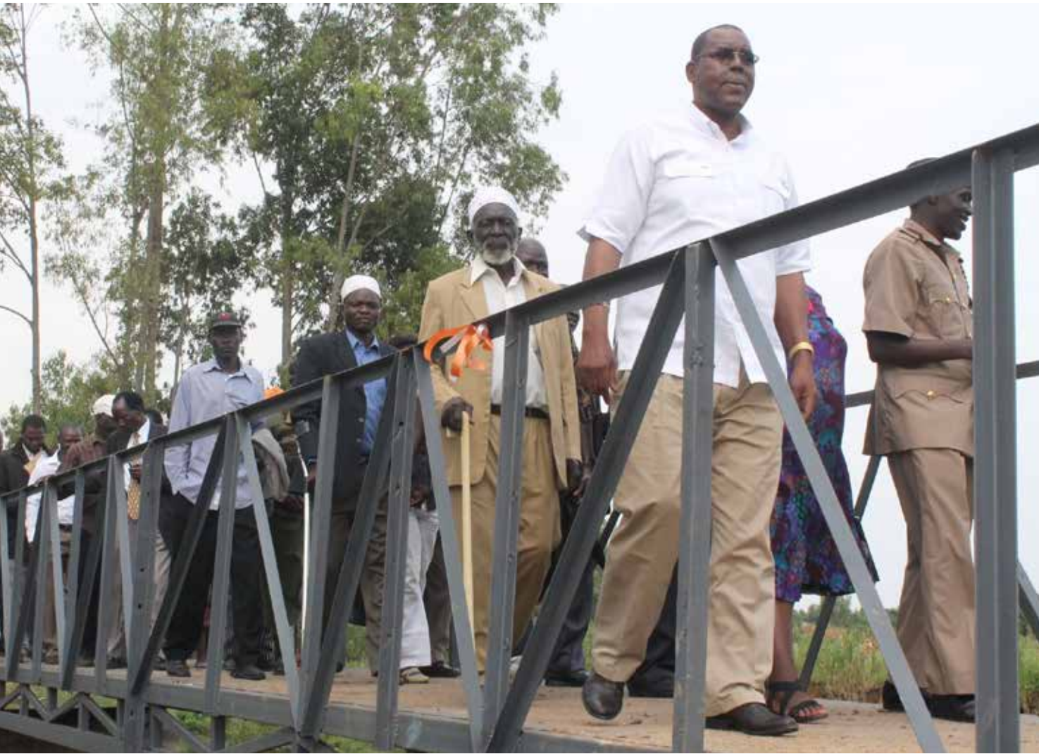
Kisumu West MP Olago Aluoch leads his constituents on a walk at Kambui-Konoka newly built bridge funded by CDF JULY 2014.
